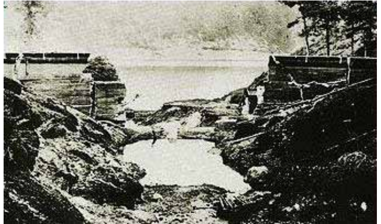
Test detonation at Nant y Gro dam (1942) Courtesy of Powys Digital History Project
