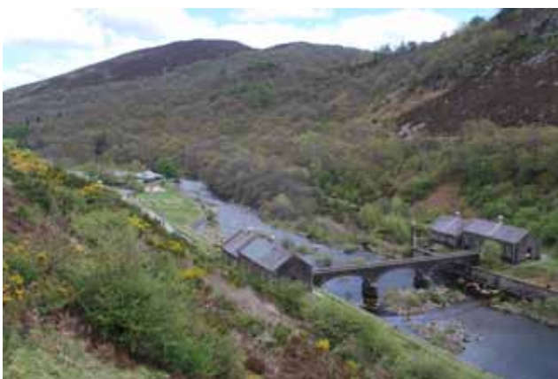
Hydro-electric plant below Caban Coch dam © Martin Haslett
