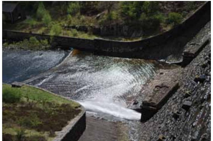
Compensation water coming out of a sluice at the bottom of Caban Coch dam © Martin Haslett
