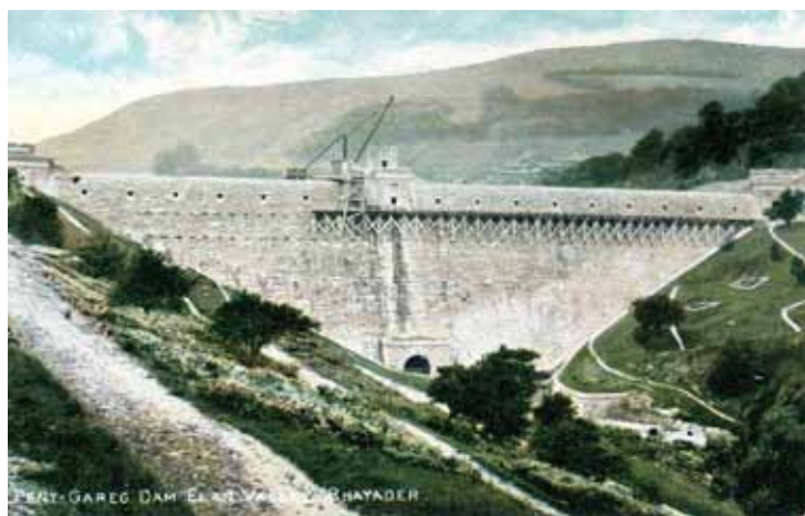
Trackway on the face of Pen y Garreg dam © Powys County Archives Office
