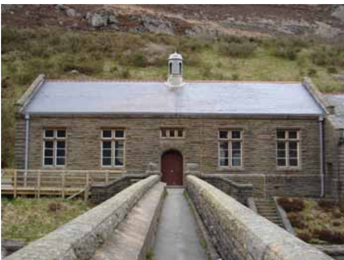
One of the turbine houses at the base of Caban Coch dam Jenny Lunn © RGS-IBG Discovering Britain
