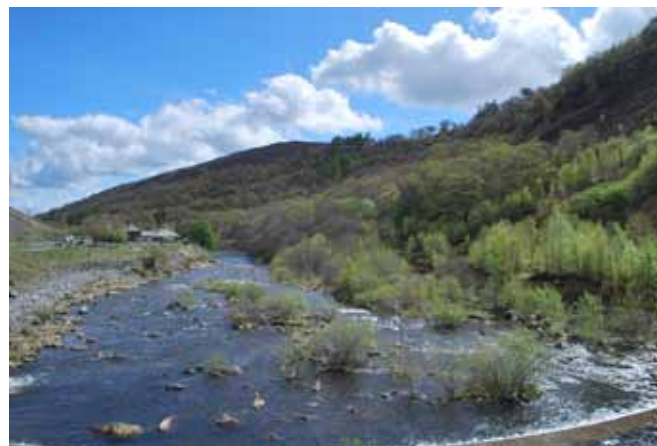
The Garreg Ddu submerged dam allows the River Elan to flow at all times © Martin Haslett
