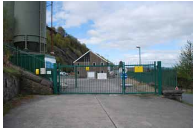
Entrance to the water treatment works © Martin Haslett
